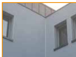
Joint de dilatation
